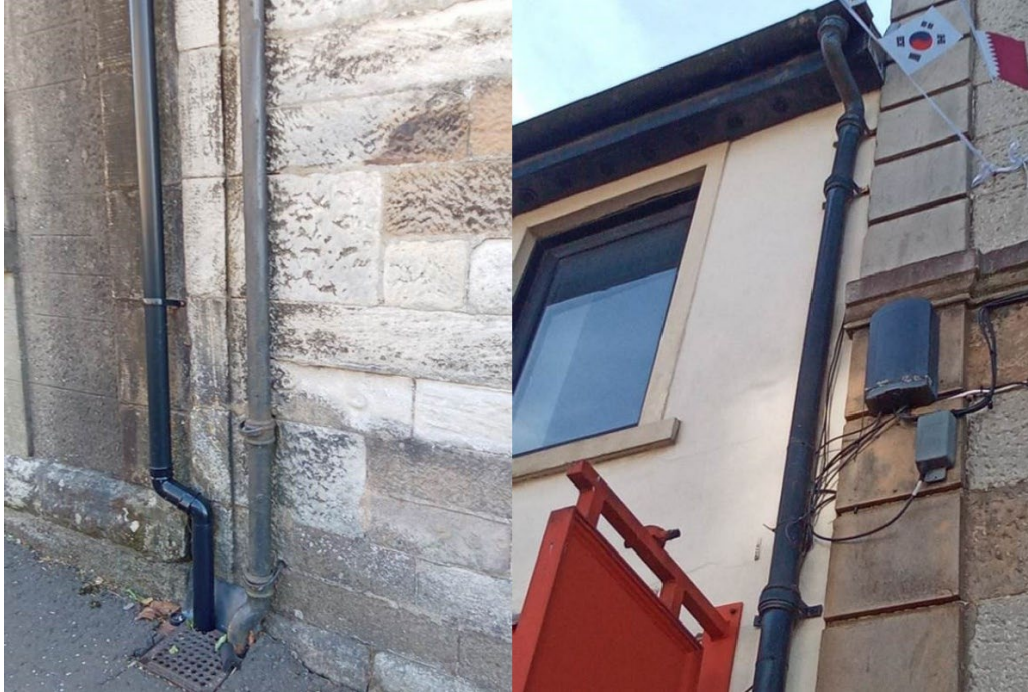
Figure 445 (Left): uPVC downpipe next to traditional cast iron downpipe (clip damaged & bottom clip missing) – poor practice in a CAA Figure 46 (Right): Traditional cast iron rainwater goods
