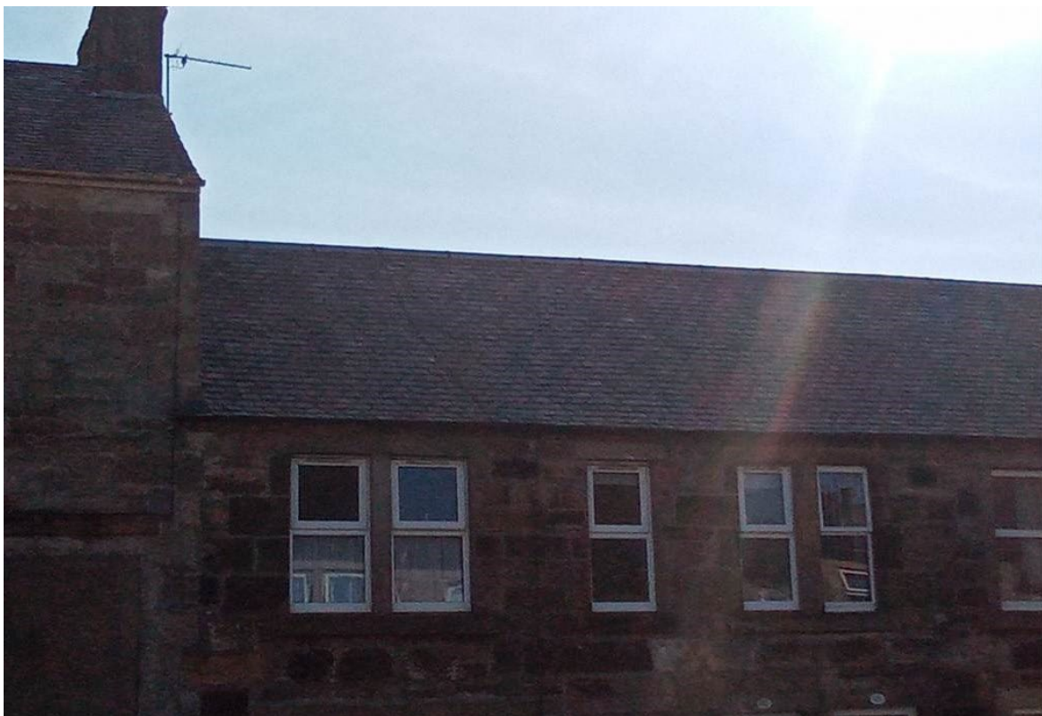
Figure 40: Traditional Natural Scottish Slate (Ballachulish Slate, distinctive in subtle muted grey tones).
