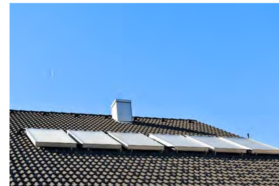
Figure 22: Flat plate collectors - fixed on the roof tiles or integrated into the roof
