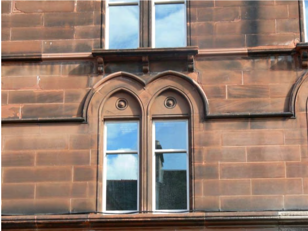
Figure 6: Appropriate restoration of windows, John Finnie Street, Kilmarnock.
