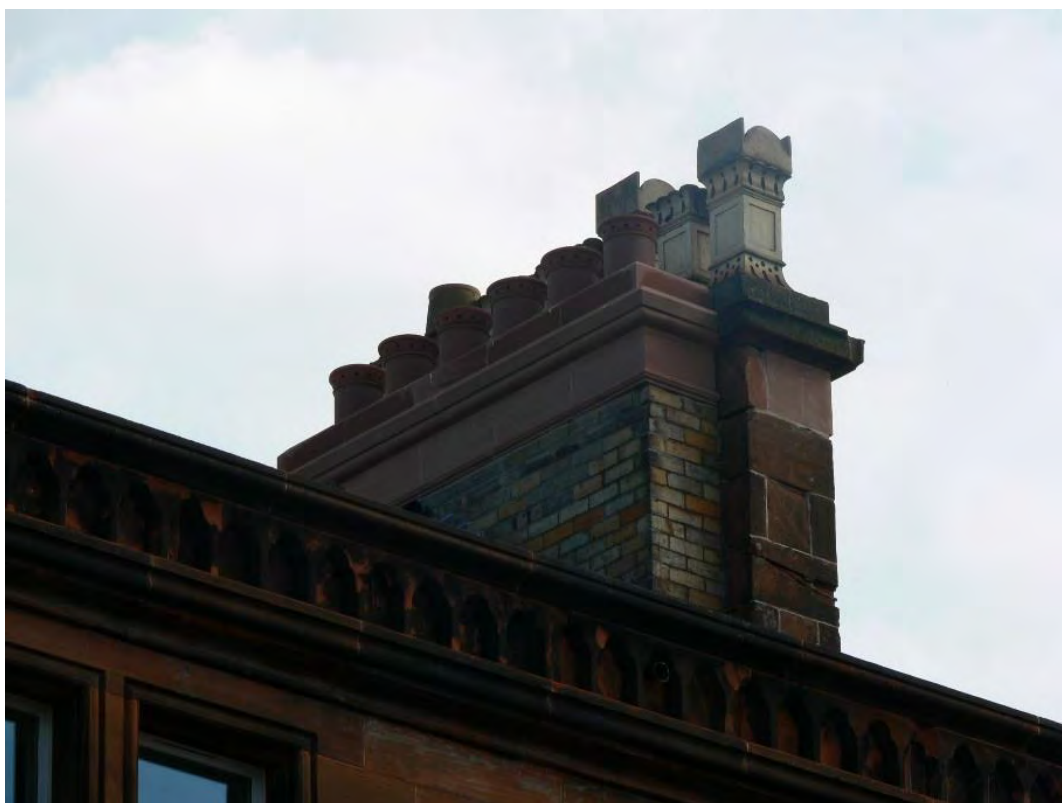
Figure 10: Appropriate chimney restoration, John Finnie Street, Kilmarnock
