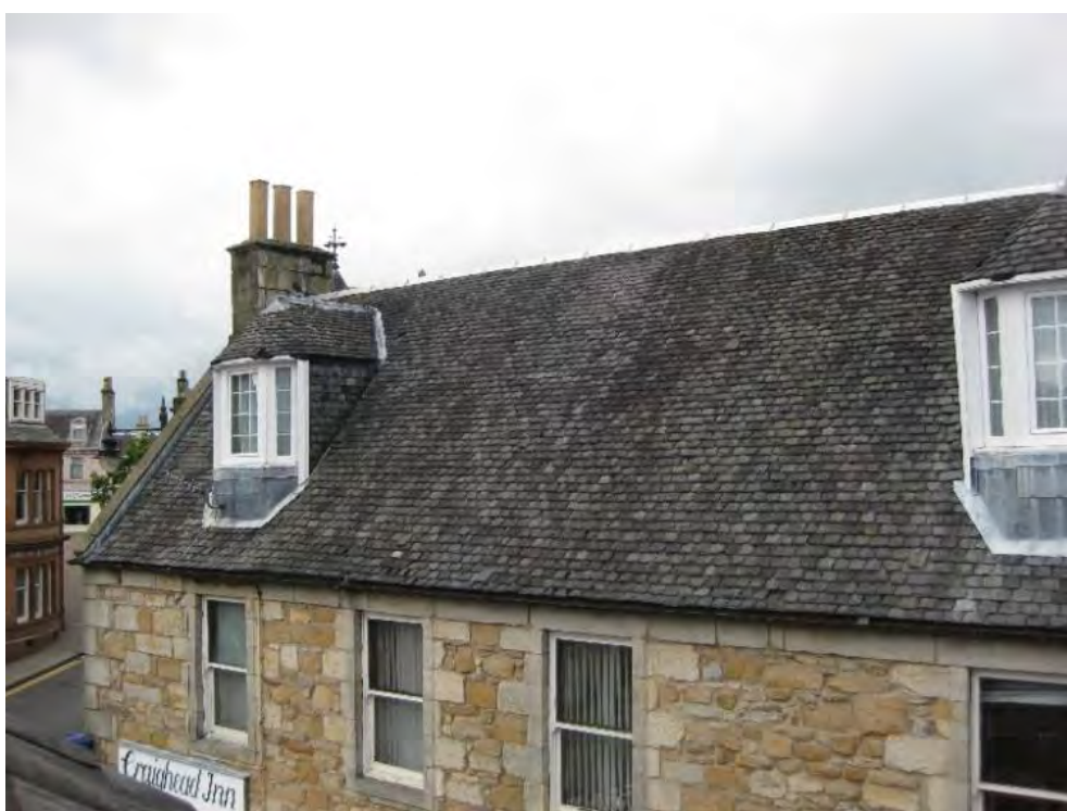
Figure 7: Appropriate restoration of a slate roof, Craighead Inn, Cumnock
