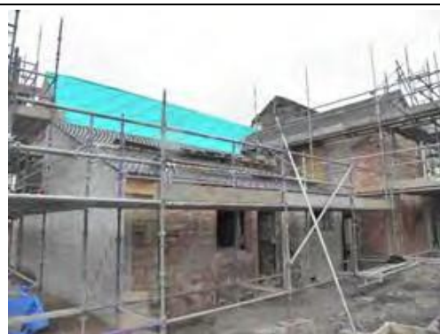
(Rear Elevation) Rear façade masonry stabilised, new pier to the right of door and installation of new steel beam & timber rafters. Roof re-slatted.
