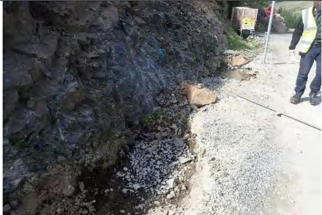
Pic 2. Unmanaged silt water identified in Audit report (Ironsides Farrar)
