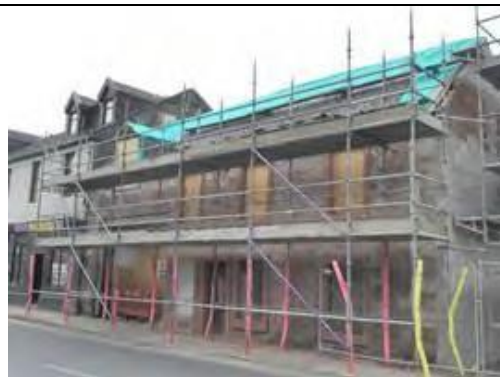
(Front Elevation) New lime mortar window bands formed. Slating to main roof pitch underway.
