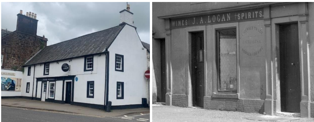
Figure 11 Although the window opening sizes have changed over time, the fascia, cornice, and pilasters remain at Poosie Nansie's
