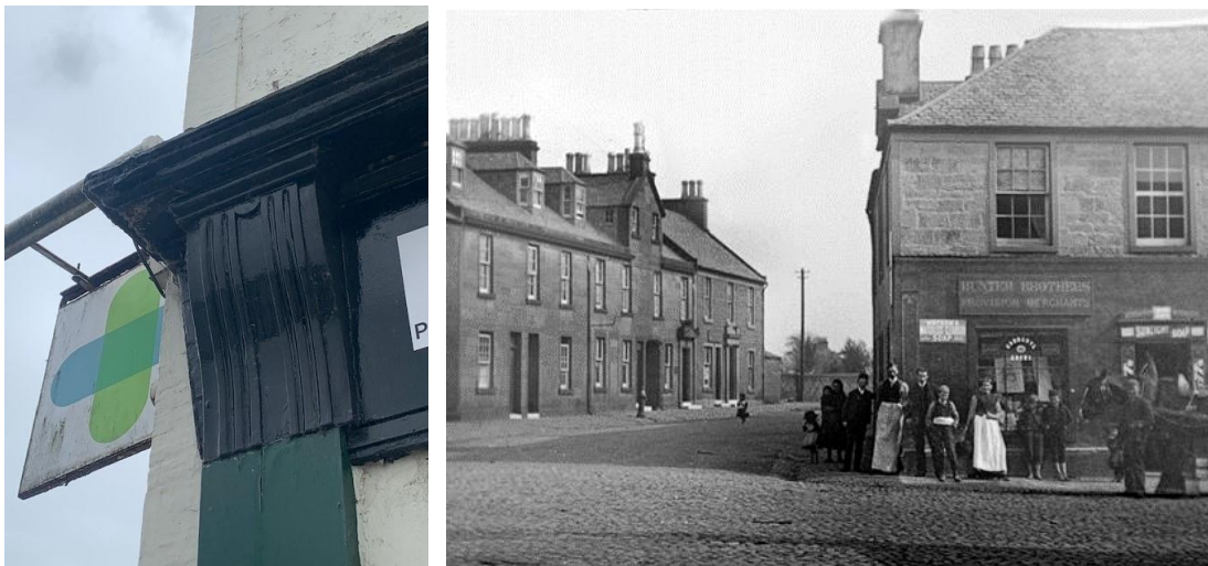
Figure 4 Console bracket at No 1 Loudoun Street. Historic photographs show however that this was a later addition to the building (refer to Gazetteer).
