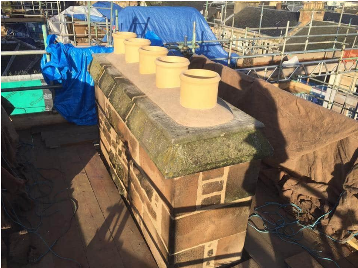
Finished haunching should look like the above
