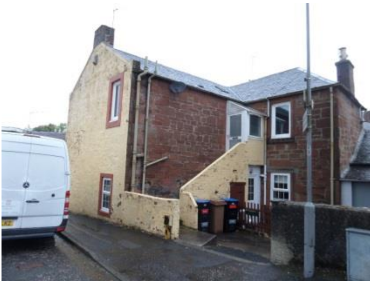
Upper floor reached by external stair
