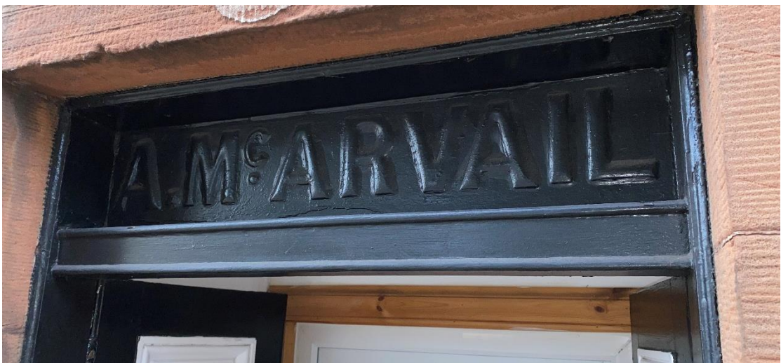
Figure 10 Evidence of the previous tenant at No 13 Loudoun Street.
