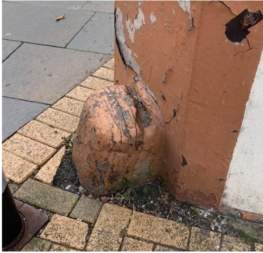
Figure 20 Corner stones and chamfered corners.
