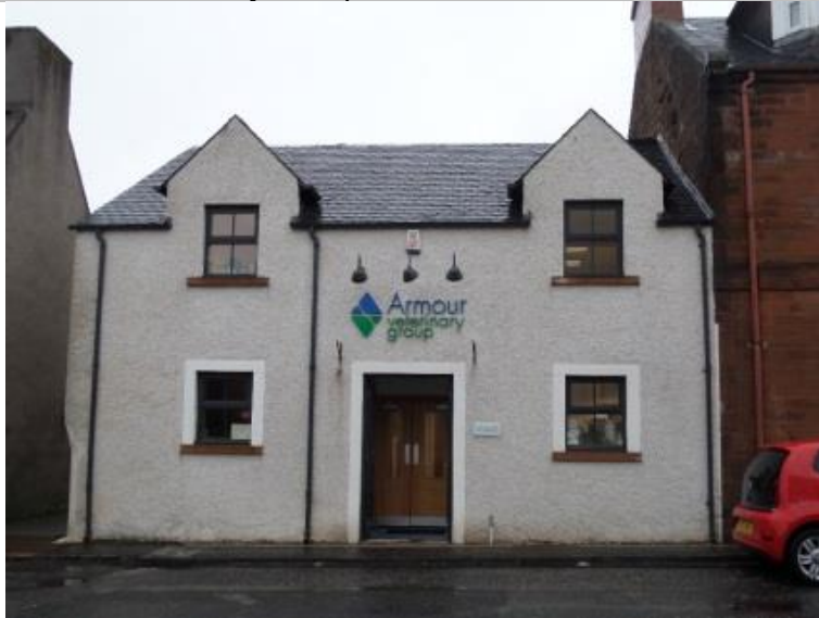
Modern building. No recommendations.
