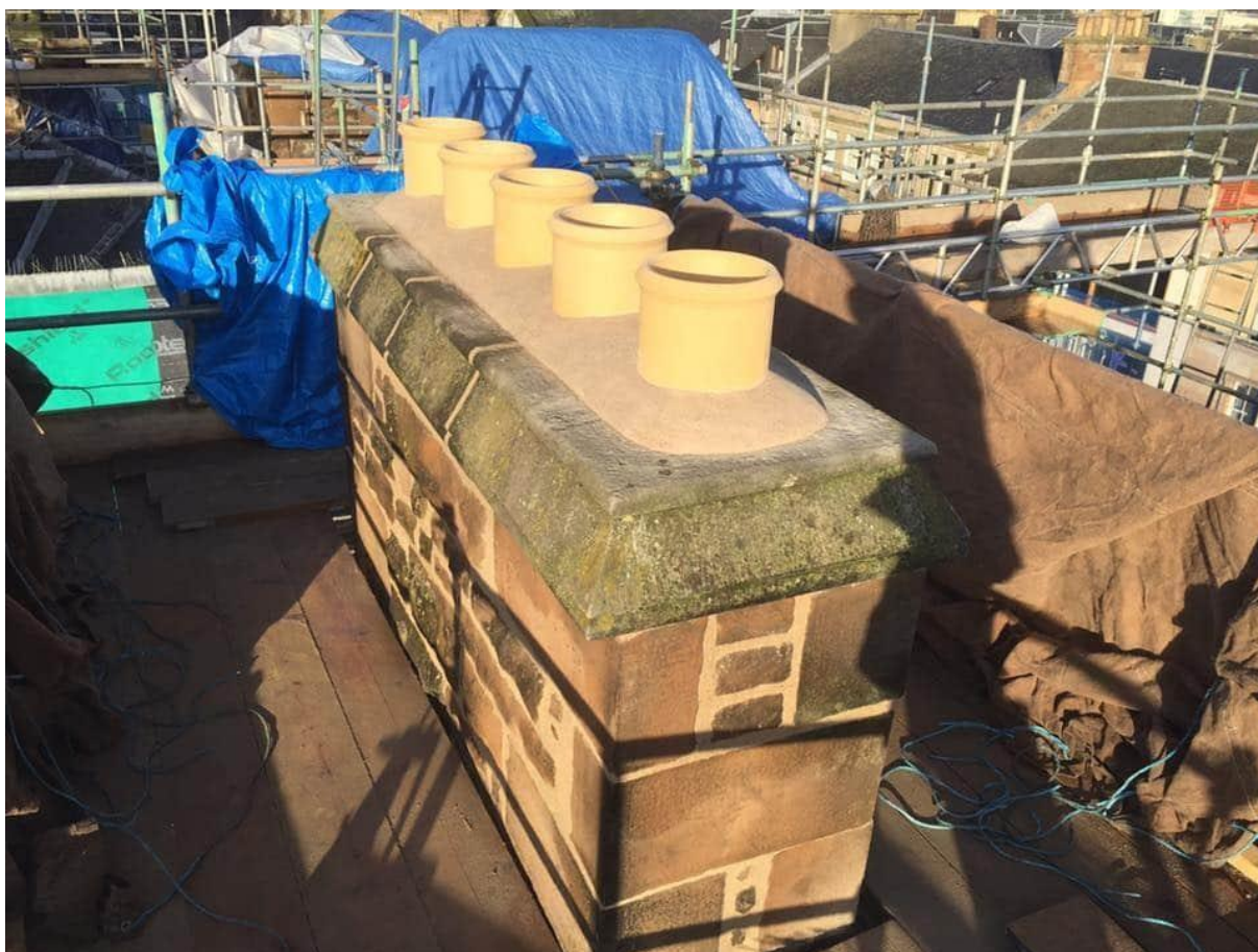
Finished haunching should look like the above
