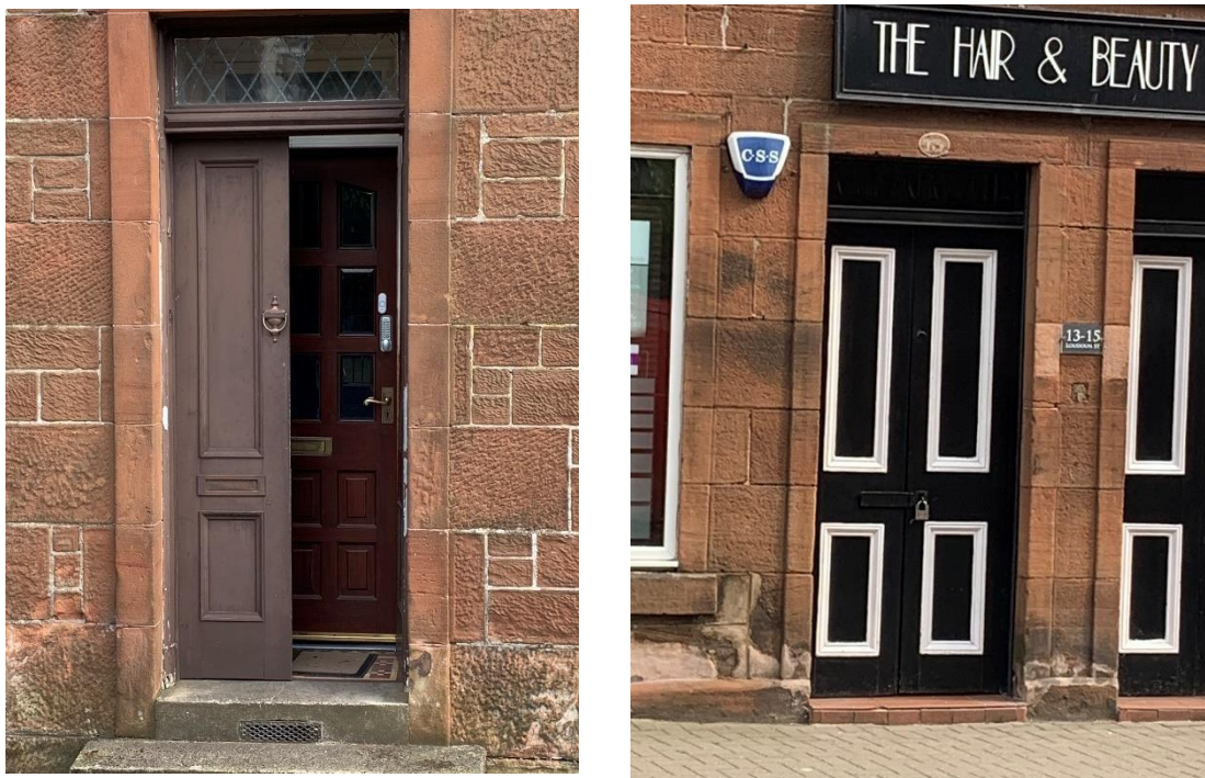
Figure 22 Storm Doors. Often with a fan light above. The double benefit of enhanced security and thermal comfort.
