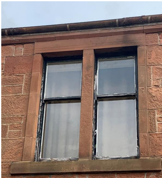
Figure 21 Timber sash and case windows
