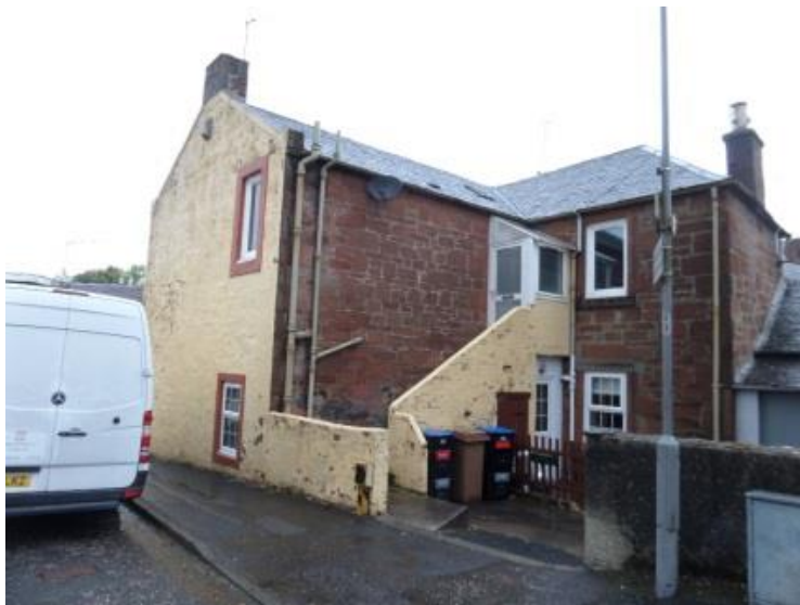
Upper floor reached by external stair
