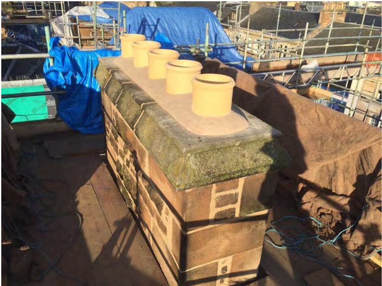
Finished haunching should look like the above
