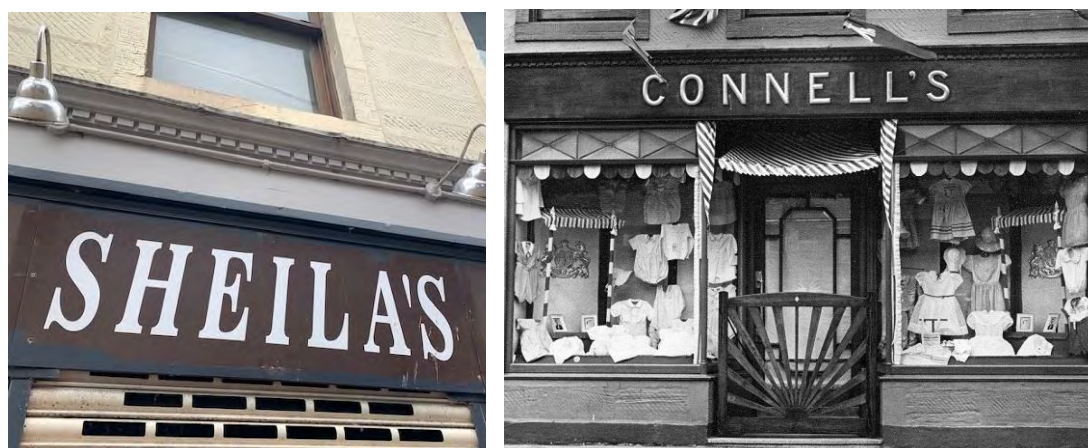
Figure 5 Dentil moulding to cornice at 9-11 Loudoun Street. Historic photographs again show that this was not original (refer to Gazetteer) but added at a later date. It is visible in the photograph of Connell's shopfront.
