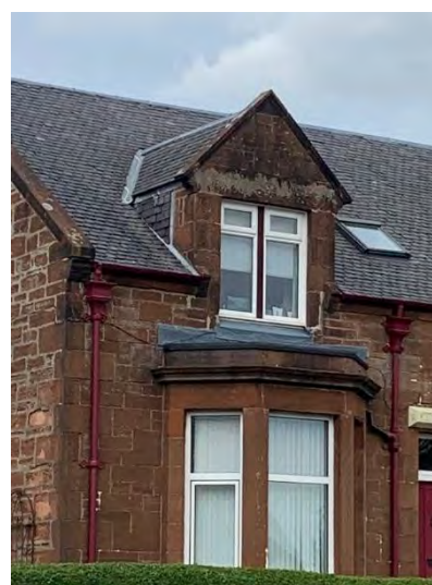
Figure 18 Cast iron rainwater goods. Decorative hoppers and wall head gutters can be found and, in some locations, decorative ear fixings can be found securing the down pipes.
