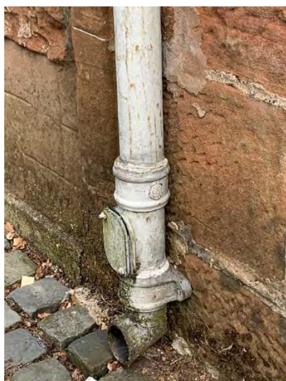
Figure 18 Cast iron rainwater goods. Decorative hoppers and wall head gutters can be found and, in some locations, decorative ear fixings can be found securing the down pipes.
