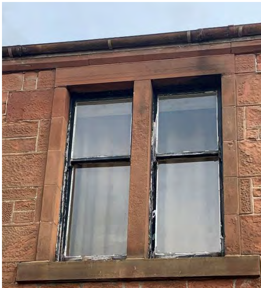
Figure 21 Timber sash and case windows
