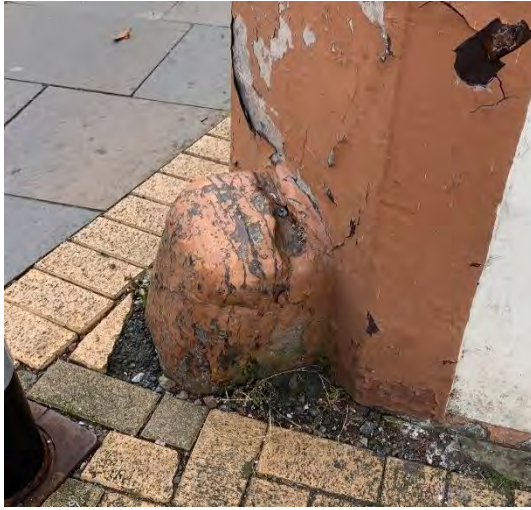
Figure 20 Corner stones and chamfered corners.
