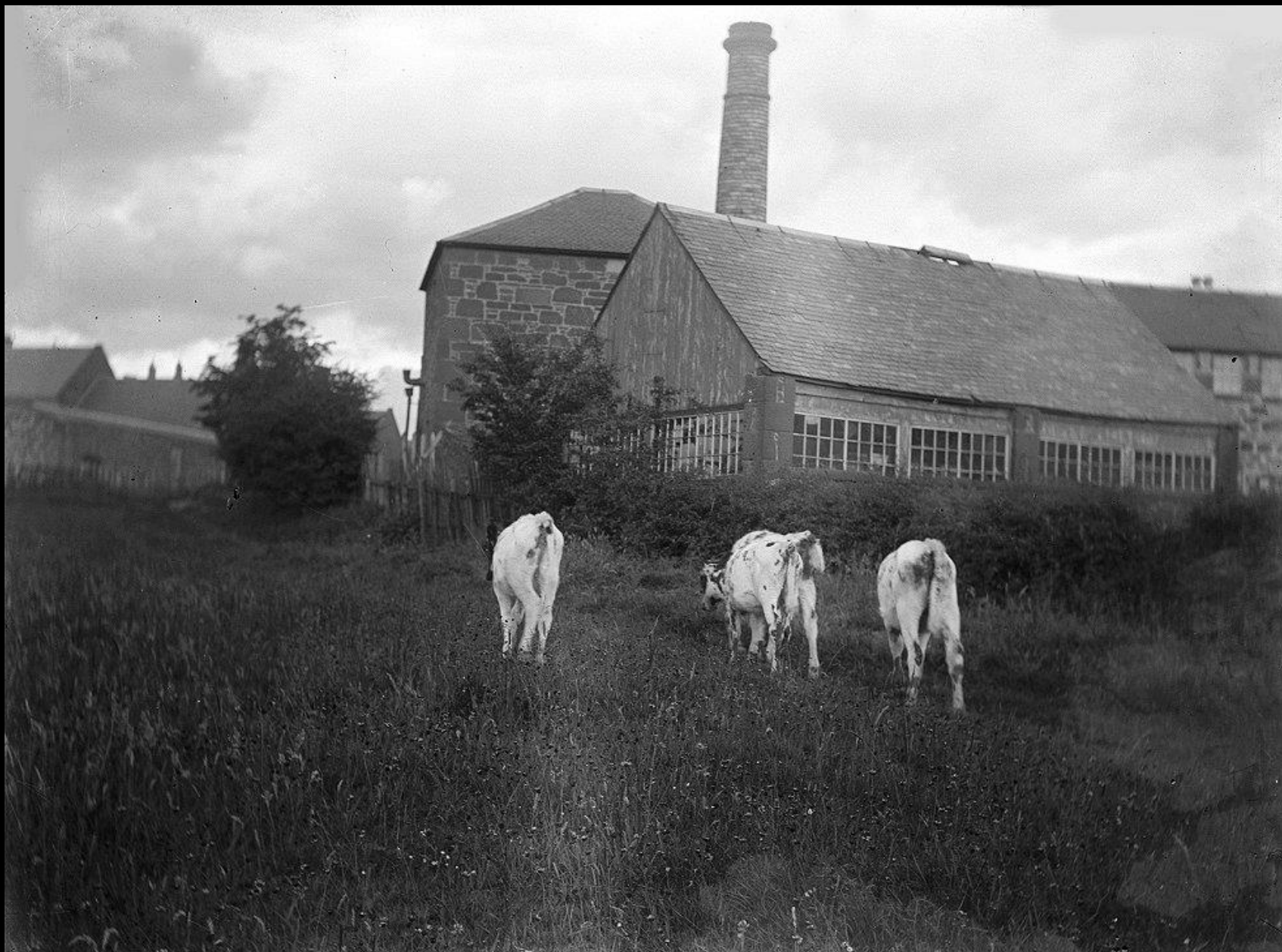
Mauchline Gasworks Chimney
