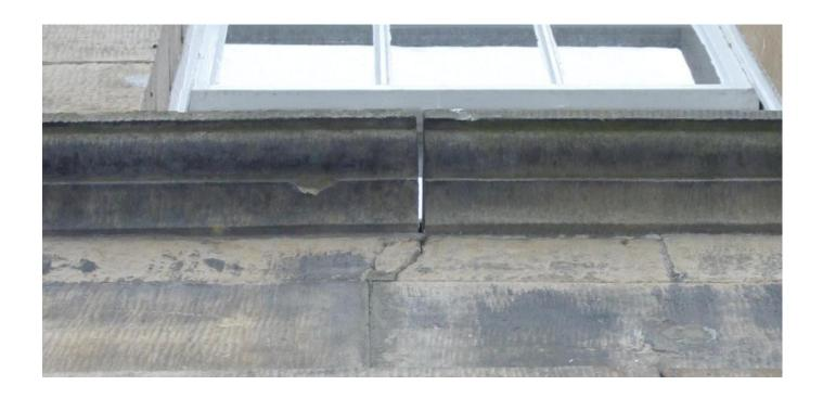
Typical open cornice joint with daylight visible through the masonry. Filling a joint such as this by hand using conventional tools is almost impossible, or so time consuming it is never properly completed in normal contracts. Resulting in incomplete work and rapid failure of the joint.
