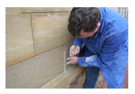
Flatten the clay strip gently ensuring it does not fill the joint.
