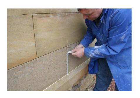
Lay it up (attach) with a flat spatula such as a small tool or better still a small wallpaper seam roller, do not press to hard, apply just enough pressure to stick unsupported to about 3/4 the way up the joint.
