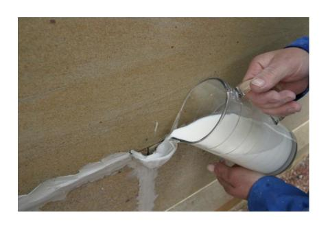
Fill at the same rate that the grout disappears into the joints...ie so the grout does not overflow
