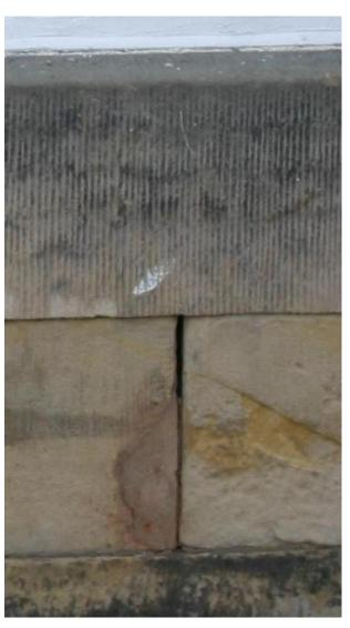
Here we can see an open joint in isolation. It is often possible to reasonably accurately calculate the theoretical maximum volume of a joint by taking height, width and depth 300mm x 5mm 100mm = 150000 cubic millimeters or 150 cubic deciliters equivalent to 150 Milliliters in liquid volume. Its would be a reasonable assumption on volume given the variation in the joint from top to bottom. This will become more relevant and clear as the next few sections unfold.
