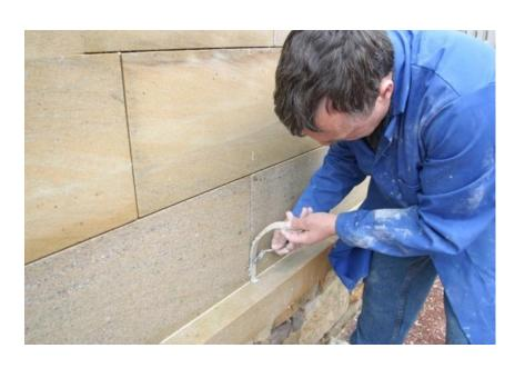
Apply the clay strip to a cleaned out joint and dampened (but not wet wall) over the centre of the joint to be grouted.
