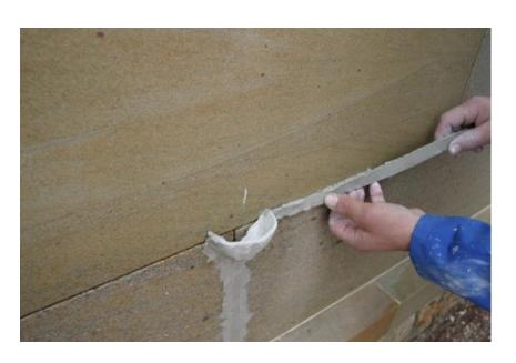
If necessary cover any open horizontal joints using clay cover strips as shown
