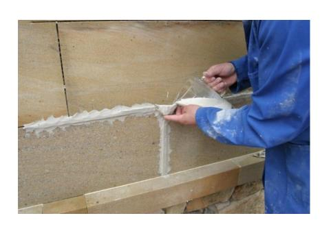
Once the target joints have been covered. Flush out the joint with water, this will readily show any areas where leaks might occur and will also give you information as to the extent of any unseen voids. If necessary, create a small weep hole at the low point of the clay, this does not replace full washing of joints before applying the clay
