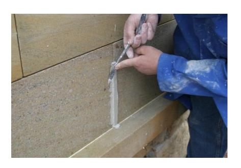
Squeeze the edges of the clay strip down to ensure there is a good bond to the stone
