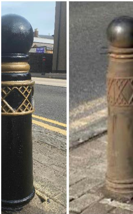
Bollard clean/ repaint 2023
