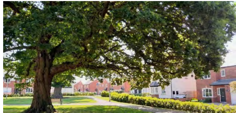
Bellway Homes' residential development Berswick Manor, Weeping Cross, Stafford (Image Source: FPCR Environment & Design)
