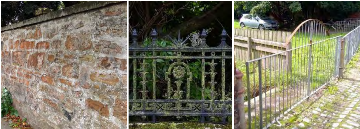
Left and centre: good quality boundary wall and railing; right: other means of enclosure of substandard appearance which illustrate their impact on the historic setting and the type of features that may be corrected through the CARS.
