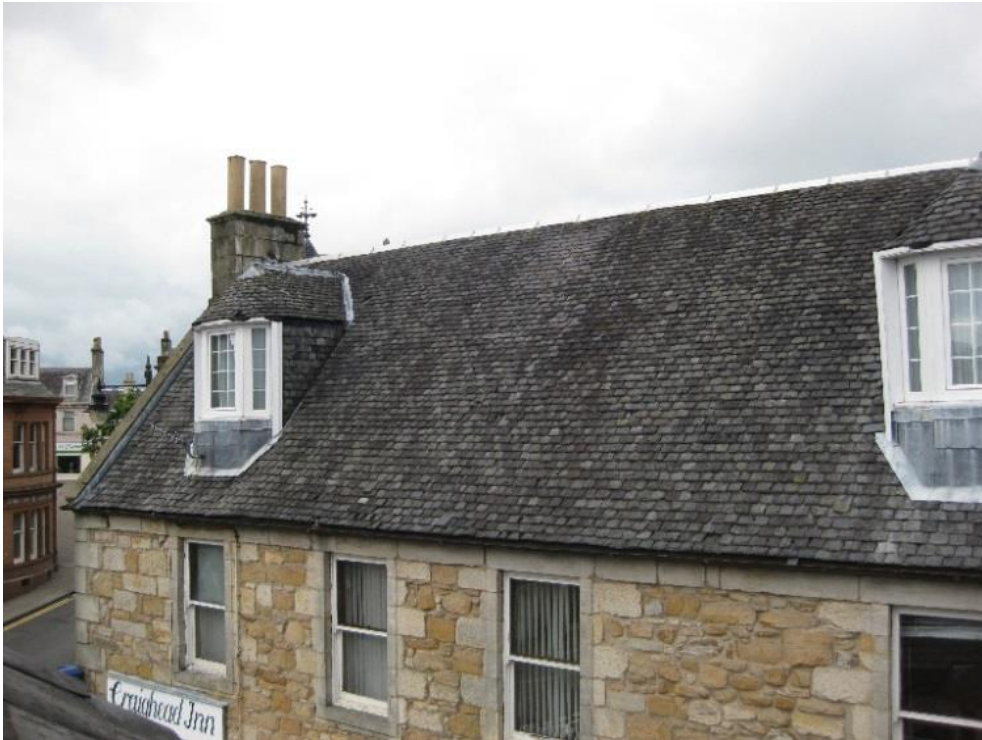
Figure 7: Appropriate restoration of a slate roof, Craighead Inn, Cumnock
