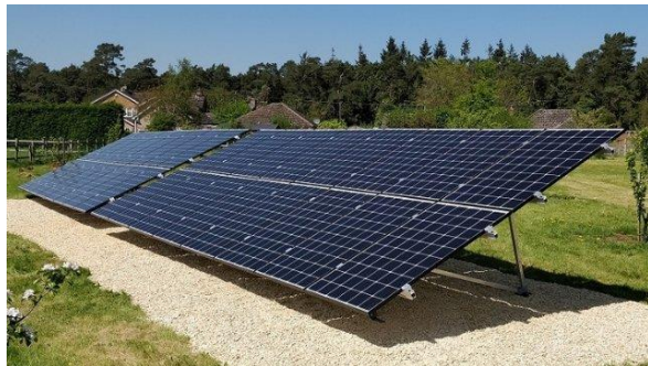
Figure 19: Ground Mounted Solar Panels
