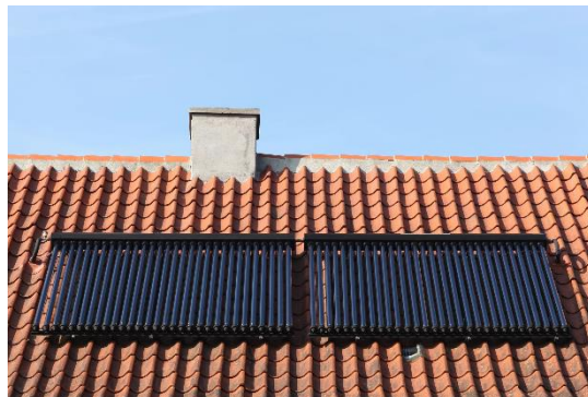
Figure 22: Evacuated Tubes - a bank of glass tubes mounted on roof tiles
