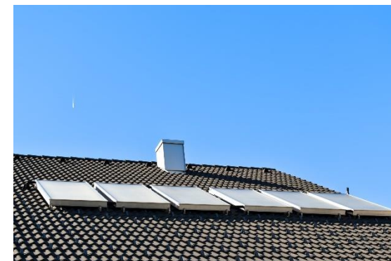
Figure 21: Flat plate collectors - fixed on the roof tiles or integrated into the roof
