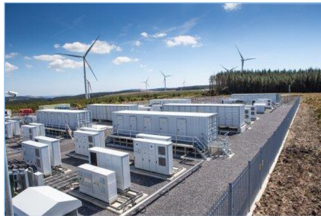
Figure 7: A 22-megawatt BESS facility is co-located at the Pen y Cymoedd wind farm in Wales.
