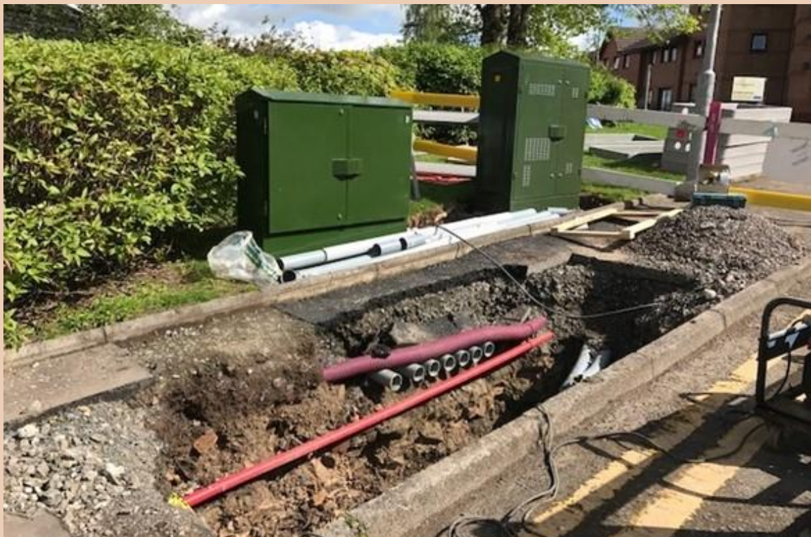
FIGURE 67. INSTALLATION OF DSSB FIBRE BROADBAND INFRASTRUCTURE
