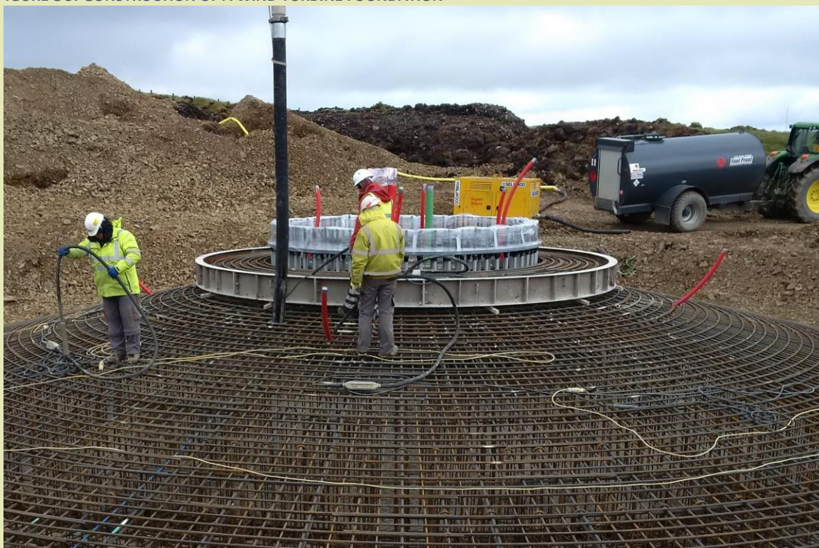
FIGURE 36. CONSTRUCTION OF A WIND TURBINE FOUNDATION
