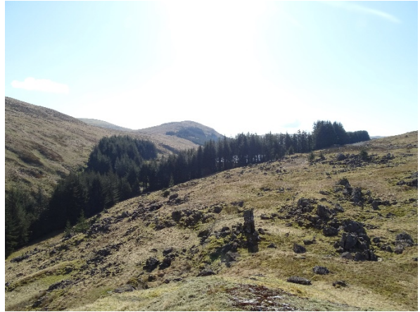
Forestry felling and OHLs at Pencloe Windfarm
