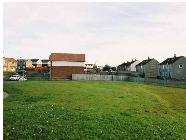
Onthank, Kilmarnock - A more unified timber edge provides the urban edge, adjacent to areas of public open space.
