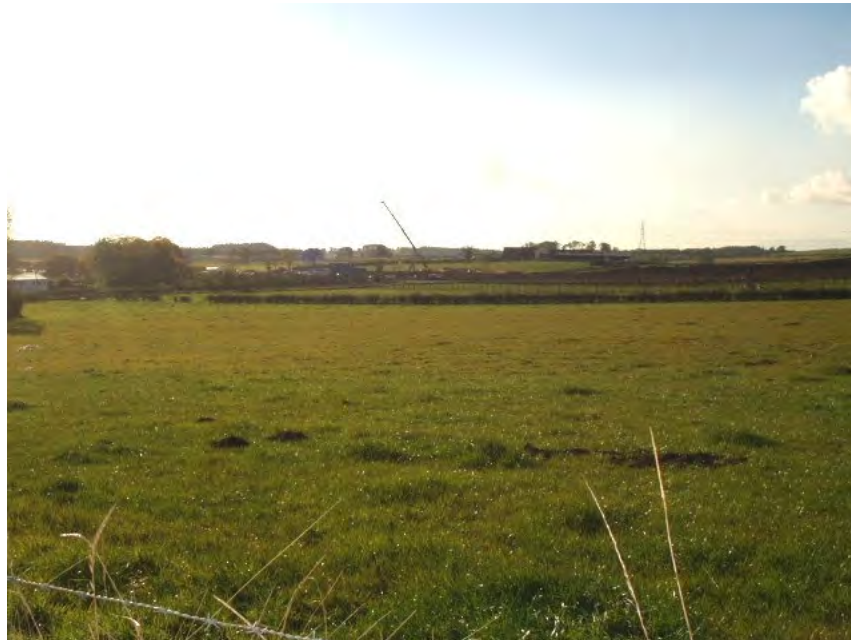
View from Fenwick looking west across A77 towards Little Fenwick, road construction underway in the foreground.
