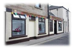
The Eglinton Hotel, Main Street, had the original sandstone facia cleaned of paint, stonework repointed and repaired and new signage installed.
