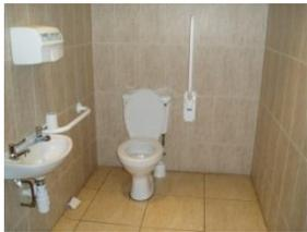
Figure 5 Insufficient Grab Rails
