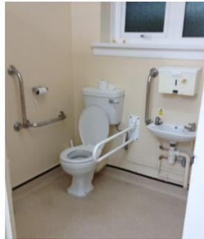
Figure 7 Sink not in correct location
