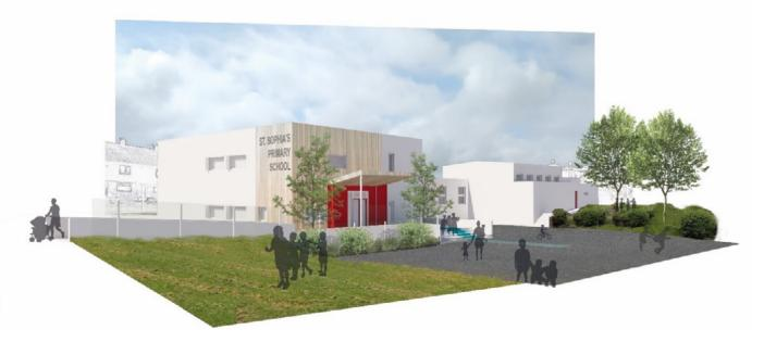
The St Sophia's Primary School project in Galston includes alterations and a deep retrofit which is being delivered to EnerPHit standards. This is a highly sustainable approach applying Passivhaus design principles of super-insulation and air tightness to existing buildings. This approach, which also incorporates a zero direct emission heating system, has the potential to reduce energy demand and carbon emissions by 75% - 90%.
