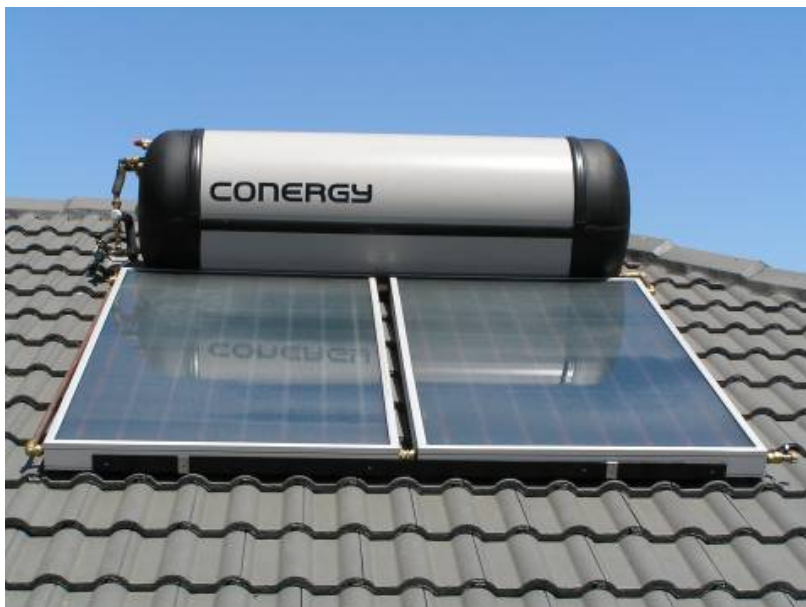
Figure 7: Solar Hot Water Installation, Energy Matters, http://www.energymatters.com.au/solar-hot-water/solar-hot-water-projects/
